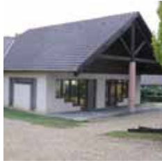
Montbonnot primary school
