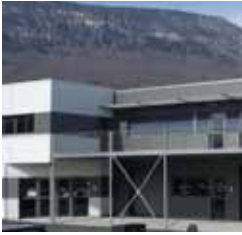
Savoie Technolac office building
